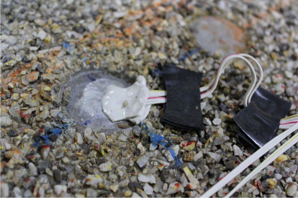
Figure 18: Installed Strain Gage
